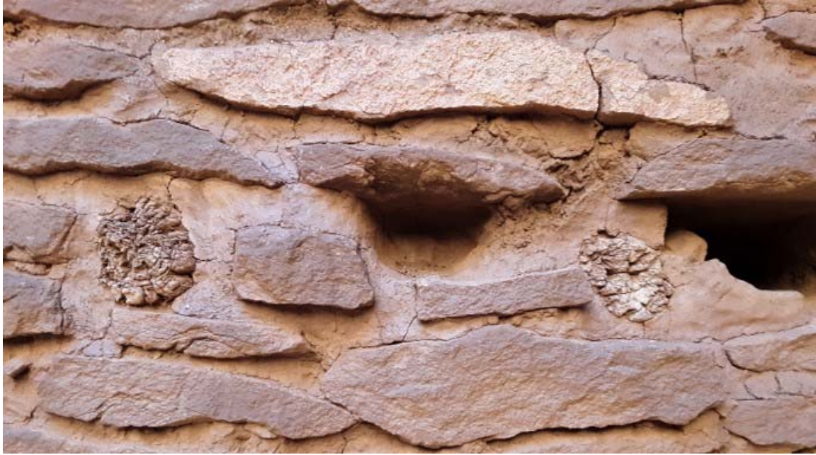
Apparent Original Wood Beam Stubbs of Upper Room Inside Wukoki Room
