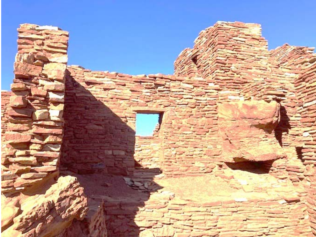
A Tall Doorway in Wupatki Pueblo Ruin
