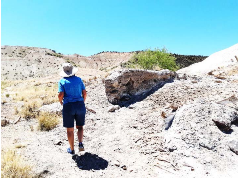
Historic Mining Operation Wall Structure at the Base of the Tailings Pile
