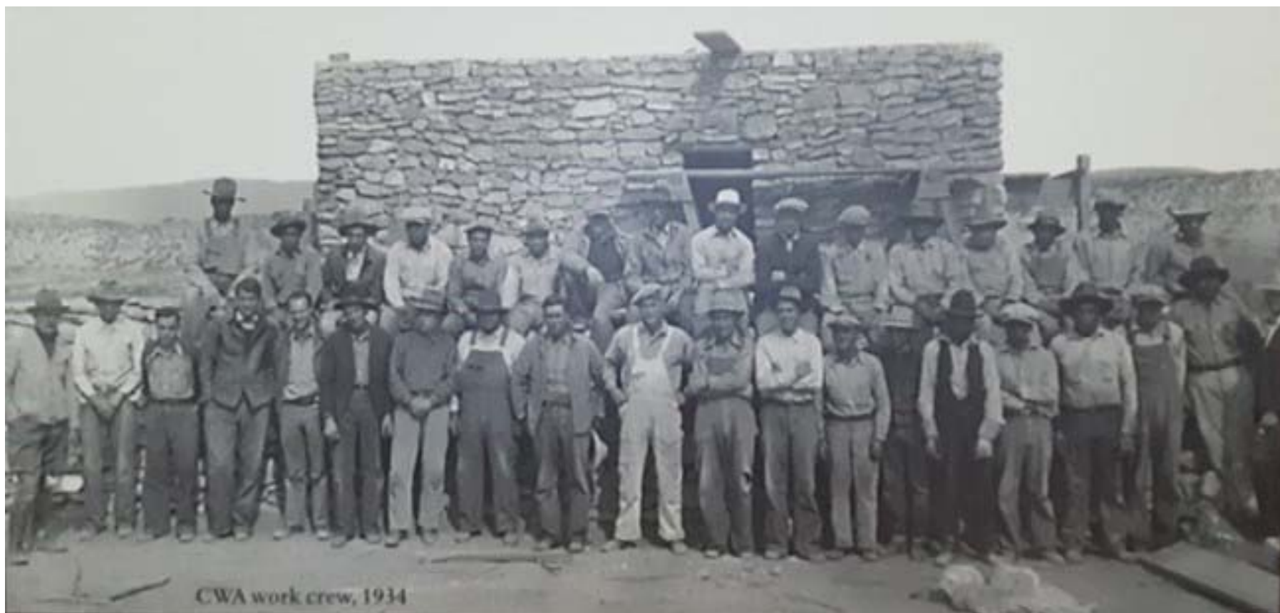
Civil Works Administration work crew, 1934. These workers did the excavation, stabilization, and restoration supervised by Archaeologists
