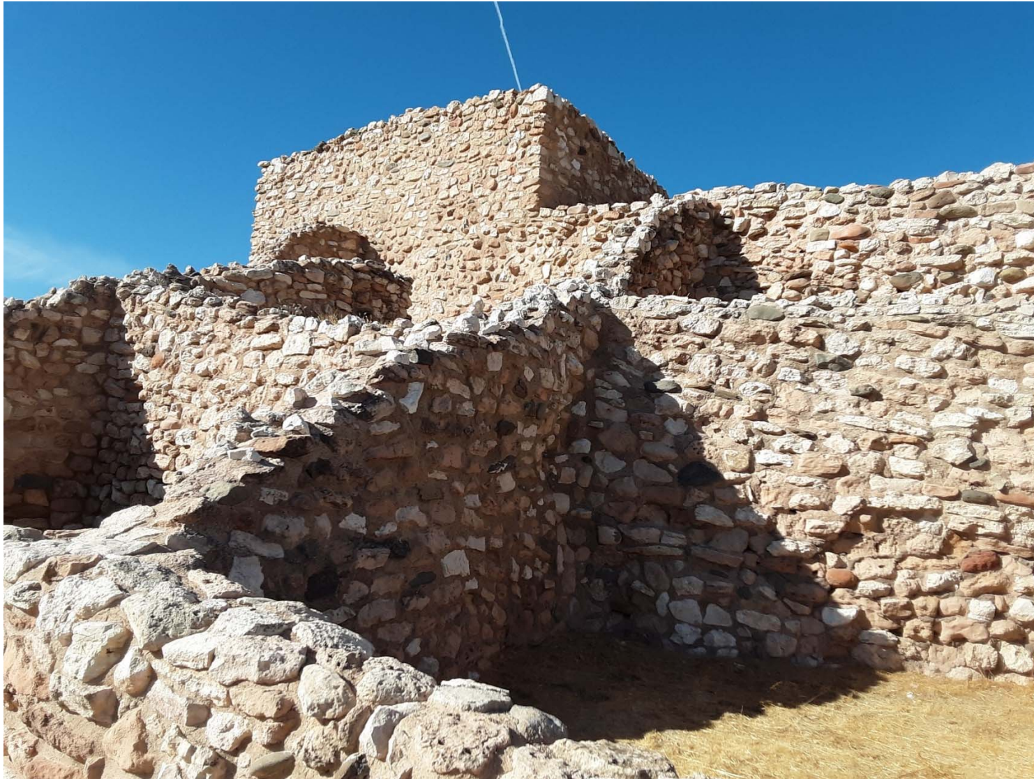
Stair step structure of Tuzigoot Pueblo. This highest part was first built on, with later rooms added stair step fashion on stair step ledges below.
