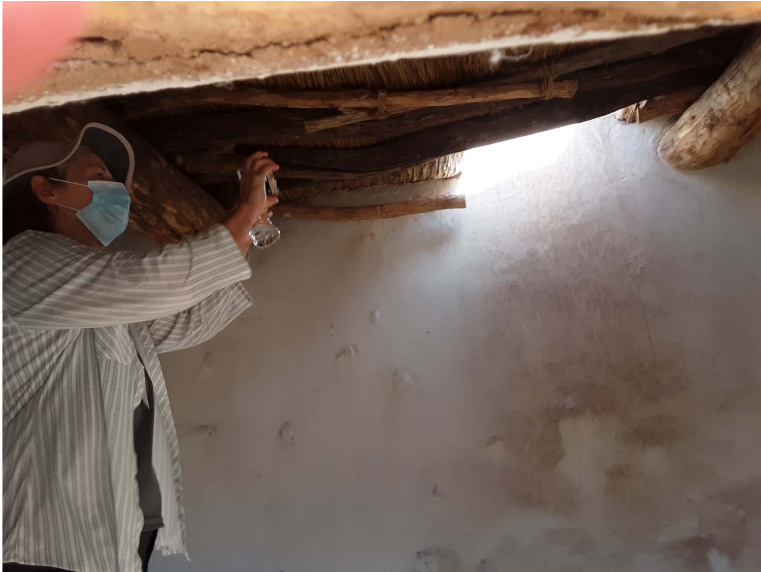
The experimental test room ceiling vent modeled after the original room
