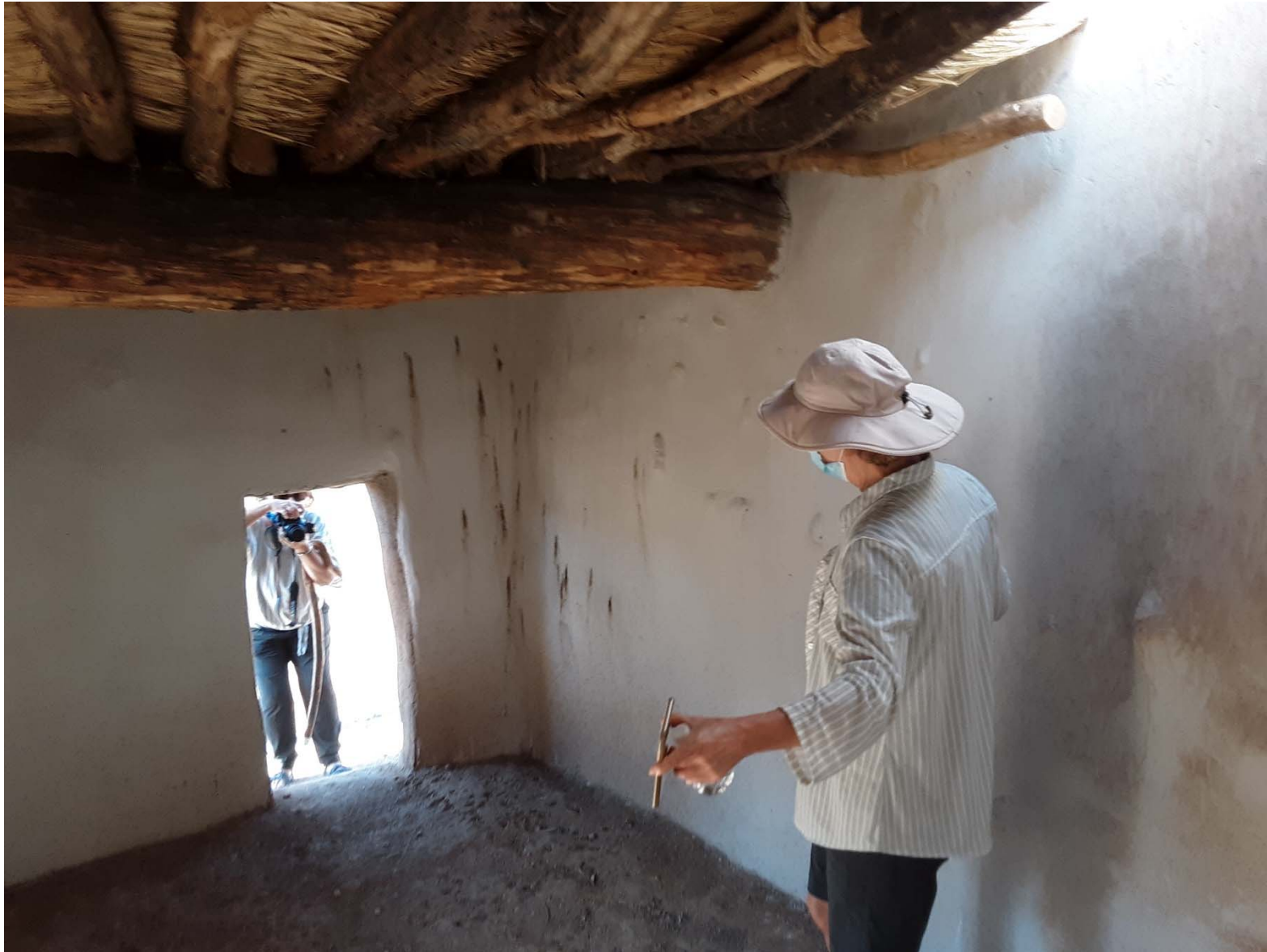
Inside the experimental test room structure
