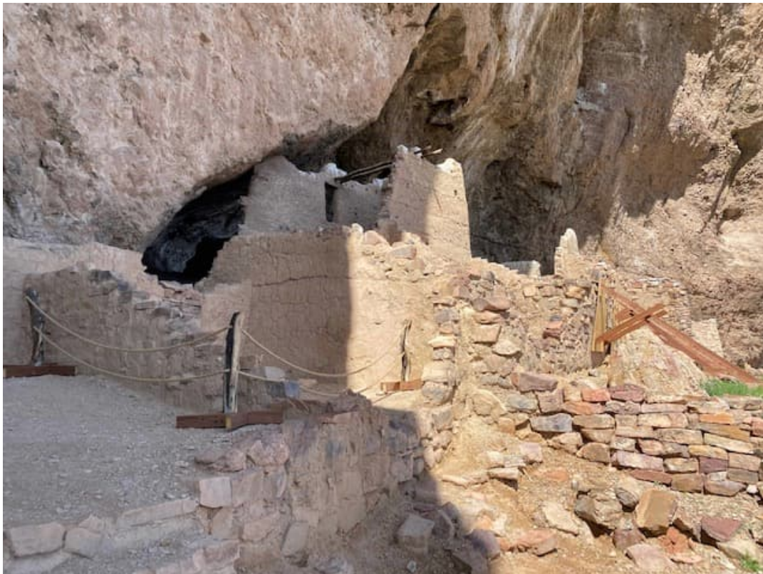
Entering Tonto Upper Ruin, Note Wooden Wall Bracing Right Center Photo by Cindie Bright
