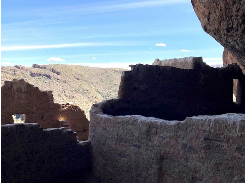
Original plaster covers most walls
