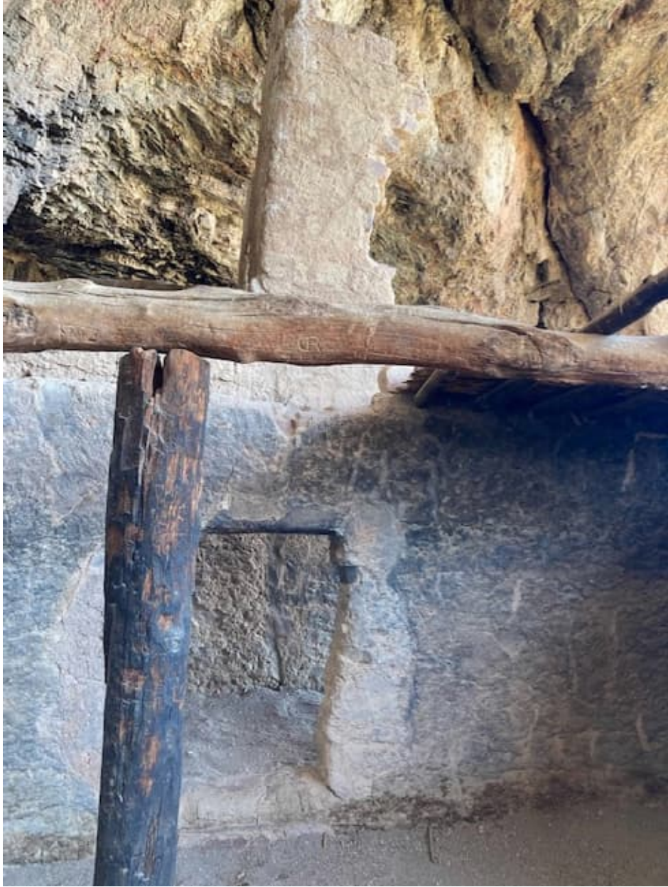
Original post & beam in the Lower Ruin Photo by Brent Reed
