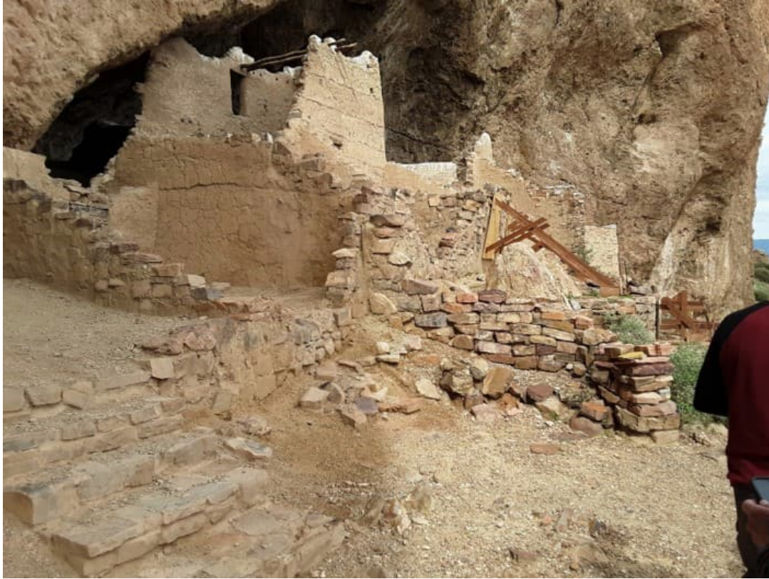
At Upper Ruin ... The steps are modern additions, as are the temporary wooden braces holding up a leaning wall center right.
