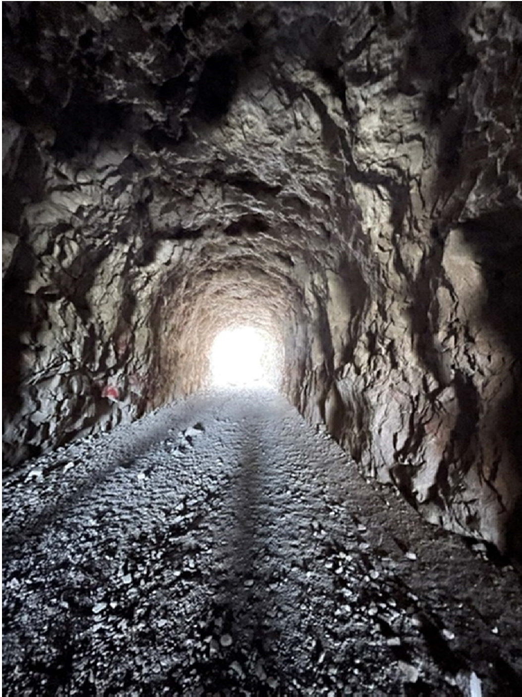
Inside the Queen Creek Tunnel
