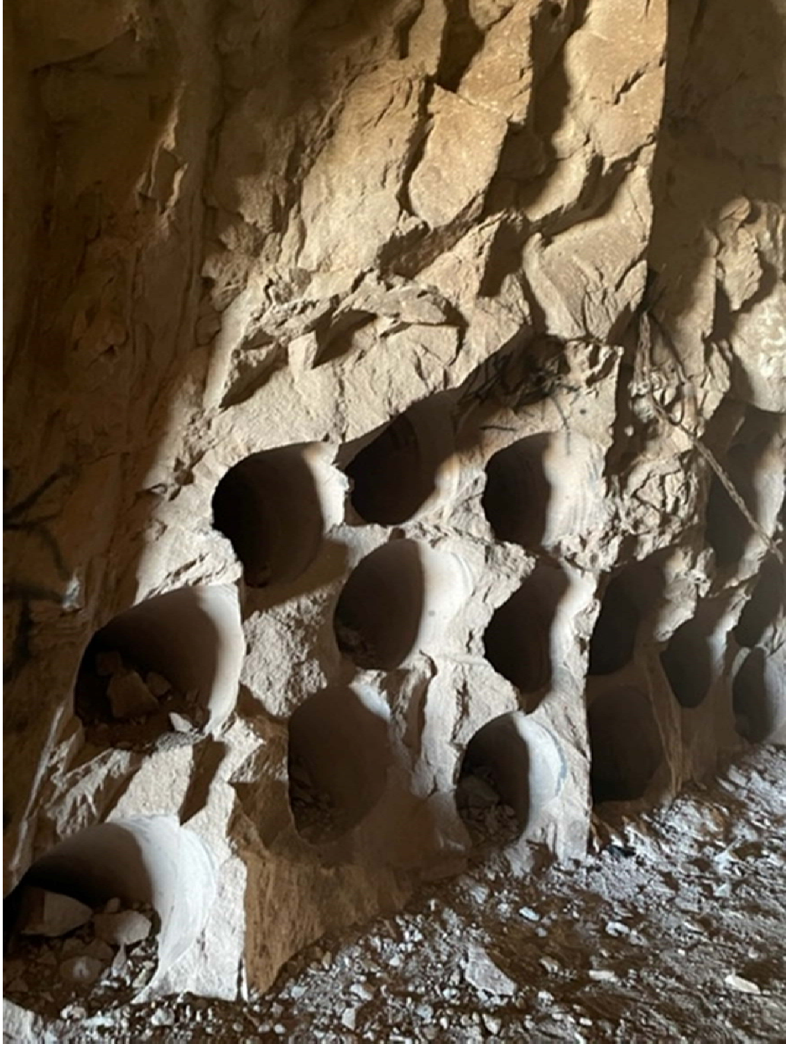
Air Vent Holes Inside the Queen Creek Tunnel
