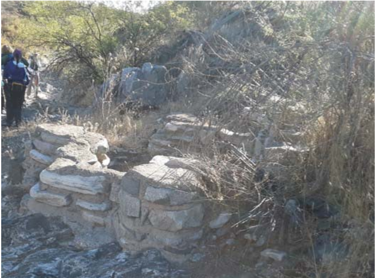
Presumed Stone and Cement Water Overflow Catchment Structure
